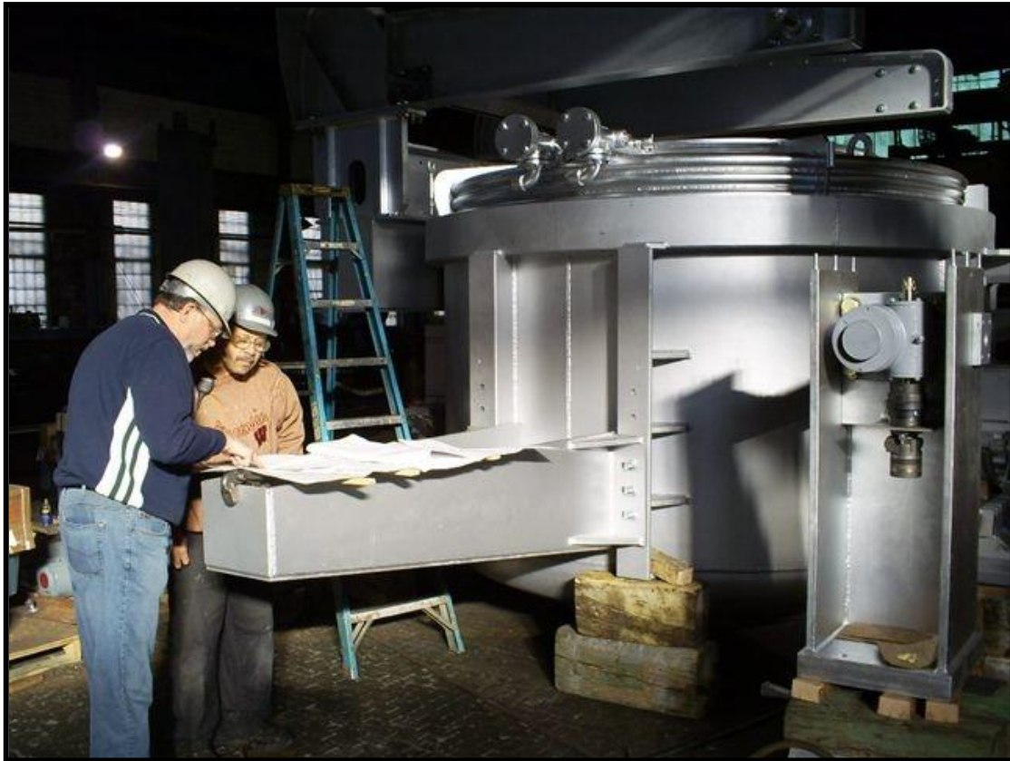
Pictured: Dan Klein and Emilio Guilbe review plans for the assembly of the Arc Furnace which will be shipped to Santiago, Chili.
